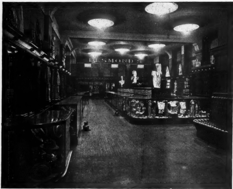
Interior lighting, by enclosed arcs, of a clothing store, Los Angeles, California.
